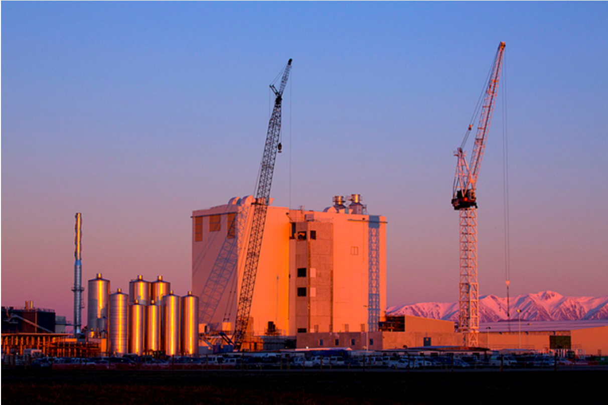
Figure 3 – Fonterra Darfield dryer 2 under construction (dryer 1 in background) image courtesy Fonterra
