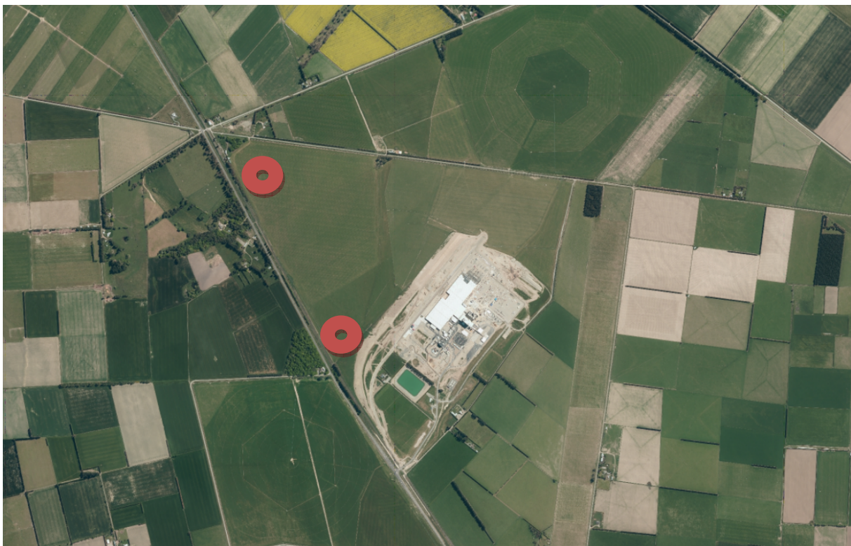
Figure 2 – Fonterra Darfield under construction with alternative locations indicated.
